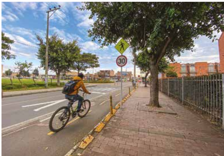
Working with the National Road Safety Agency on a pilot project, the Automobile Club of Colombia's SR4S assessments are resulting in upgraded infrastructure.
